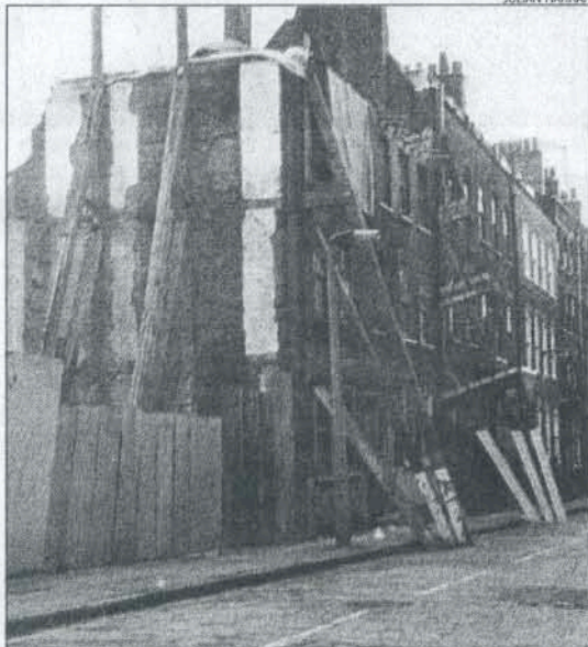
No. 5's demolition in 1977 was halted by conservationists
